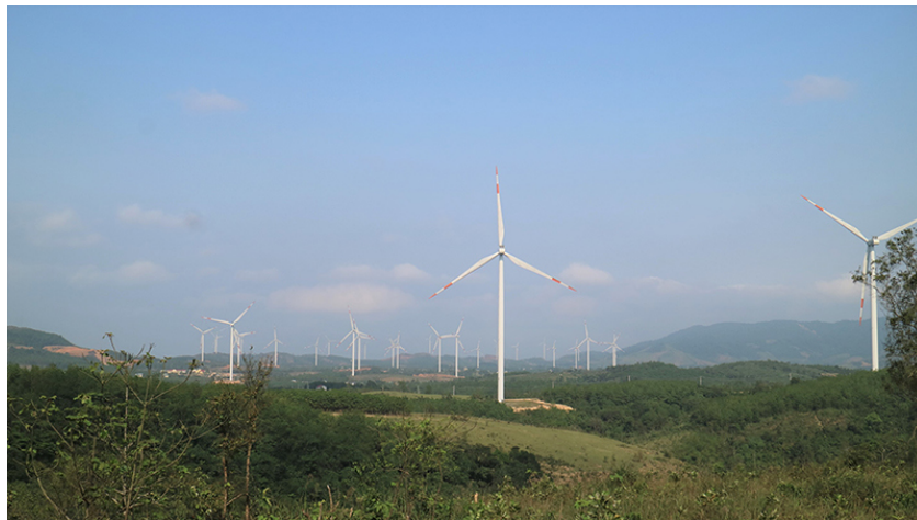
A wind power project in Quang Tri Province. Photo: Minh Trang/VGP
